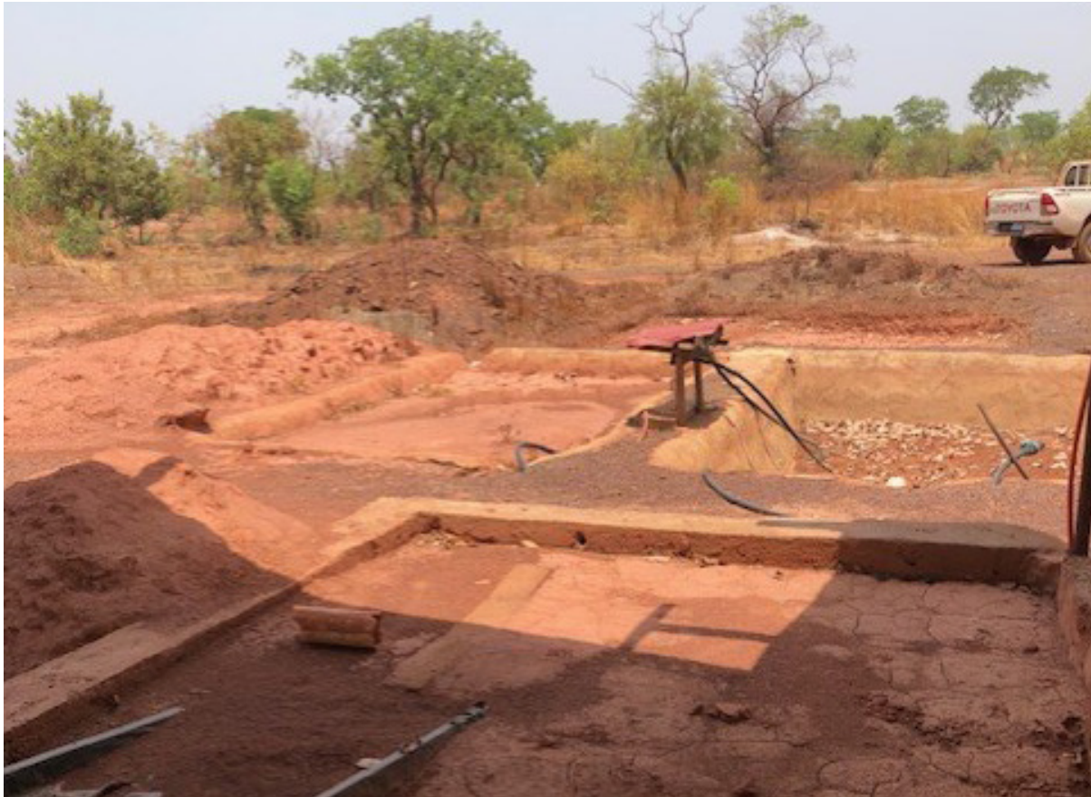
FIGURE C1. A full settling pond in Guinea
